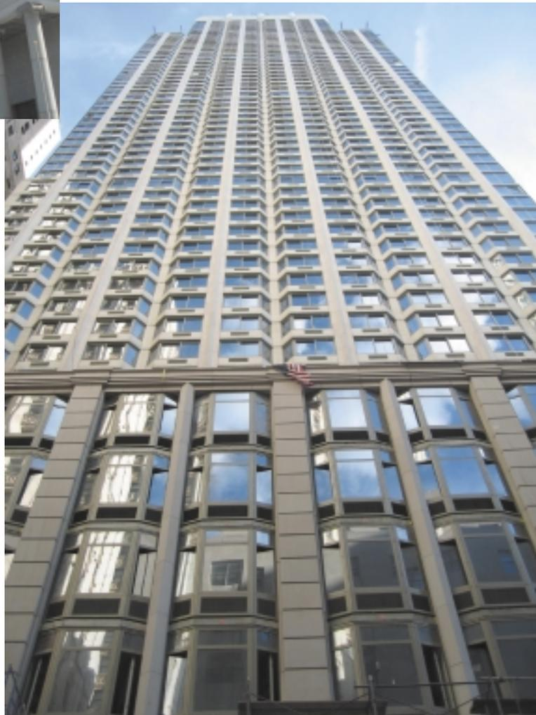
*The lightweight StoneLite® panels made it possible to incorporate natural stone cladding on the exterior of even upper levels of Barclay Tower.*
