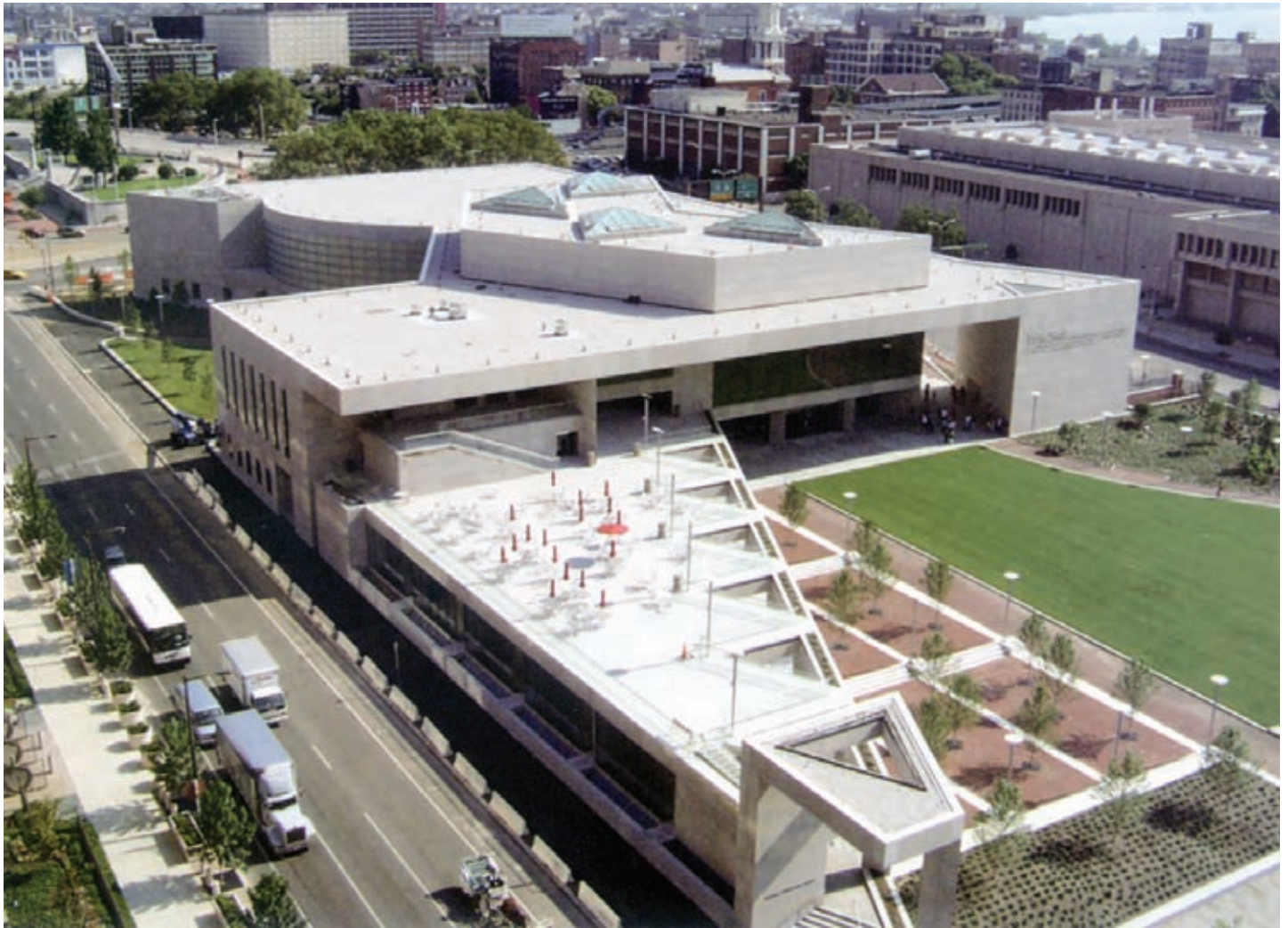
Pei Cobb Freed & Partners' design team investigated a number of Stone Panels' installations before specifying 9,000 square feet of StoneLite® panels for exterior walls over the atrium.
